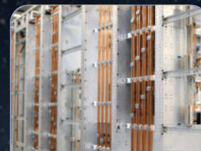
Inter-Connection Link Work
