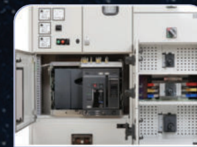
Feeder Link Work
